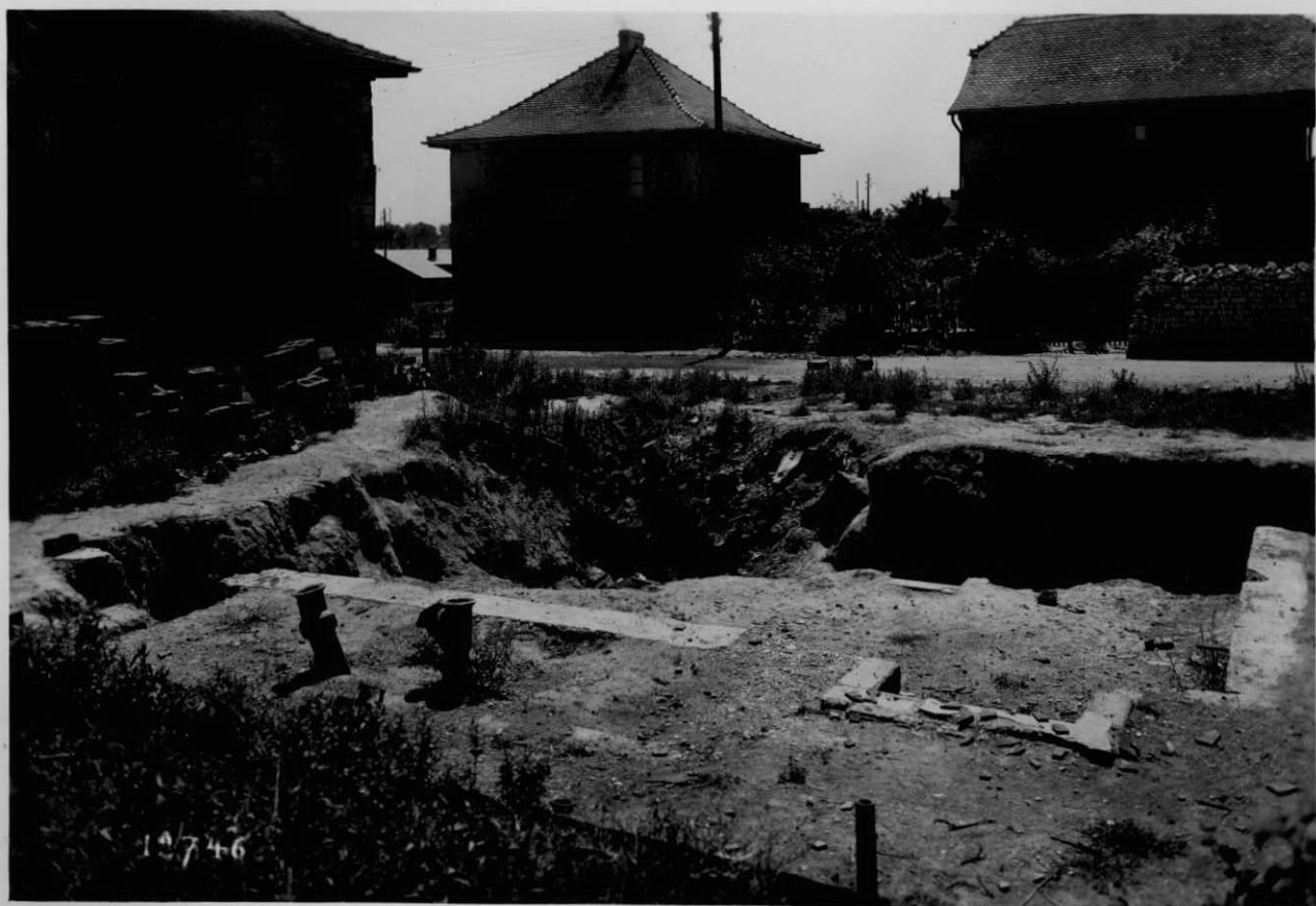
Segment of 63 View of the structure from the south
