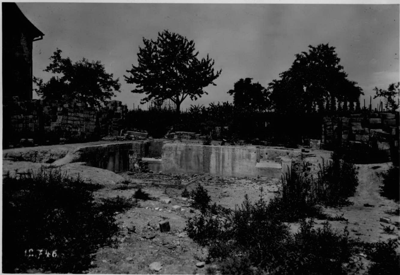
Segment of 63 View of the structure from the north
